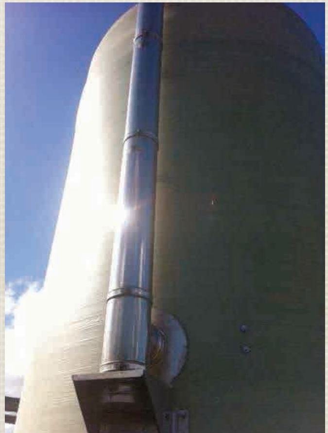
10 tonne fuel store and 200mm twin wall stainless steel flue
