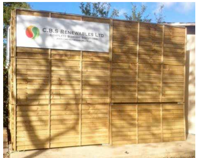
8 tonne Fuel Store with wood cladding
