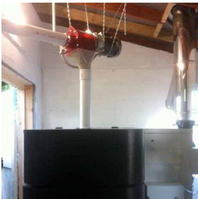
Auger-Fed to 199kW E-COMPACT Pellet Boiler
